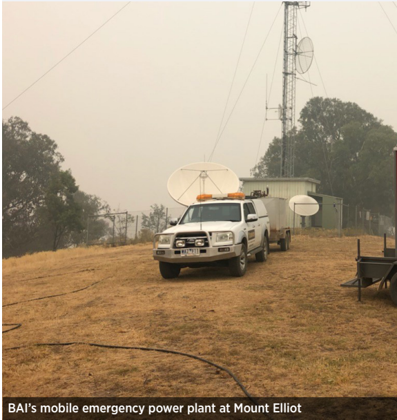
BAI's mobile emergency power plant at Mount Elliot
